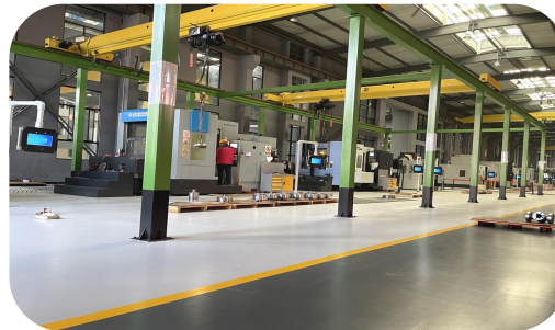
Industrial electrical equipment
